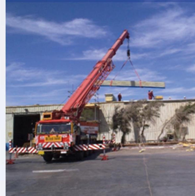
~ Project of complete installation for steel structure building in sugar factory. The works include fabrication, welding and erection works for all the steel structure parts.
